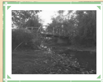
Speaker Road Bridge
