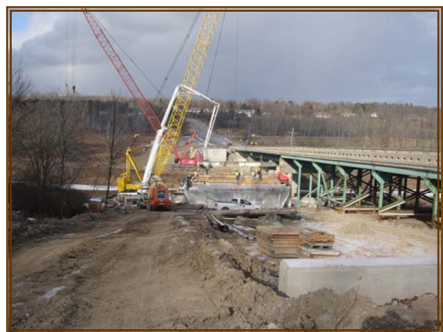
Wadhams Road Bridge over the Black River
