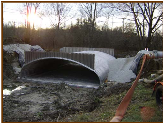
Palms Road Culvert
